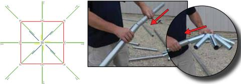
3. Take the combined hip rafter poles (Green/HT2GST80) and slide onto the remaining post slots on the 8 way crown (F048WCHT). Lining up the holes until the push pins engage.
