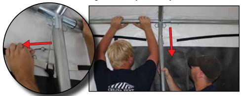
7. On one side remove both legs with base plates from the corners, place off to the side, and carefully set the frame down. *NOTE: Do not set frame*
