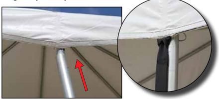
13. Locate the remaining tent top straps, 120" (300 cm) in length, and attach. Attach the loop end through the 1½" (3.81 cm) welded D ring, run the rest of the strap through the loop and outside slot of the base plate, and pull tight.
