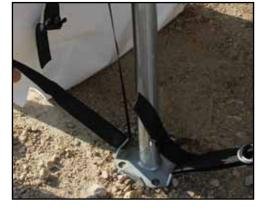
18. NOTE: Center tent top before tightening all straps by centering the patch with the 8 way crown. Tighten each strap by running the tail end of the strap through both D rings and then back through the lower D ring. Pull the tail end downward to tighten. Use a foot if necessary to tighten the
