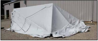
8. Remove the other two corner legs and base plates, place off to the side, and carefully set the frame all the way down. *NOTE: Do not set frame on sidewalls*.
