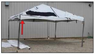
12. Put the other four legs with base plates on the bottom of all of the side tee fittings and pin with pin & bail.
