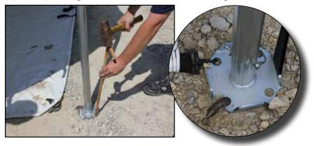
17. Take the ends of the straps down through the outside slot on each base
