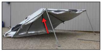
10. Locate the corner tent top straps, 120" (300 cm) in length (HT531). To attach the tent top strap on a corner take the loop end through both  $1\frac{1}{2}$ " (3.81 cm) welded D rings on each side, run the rest of the strap through the loop, and pull tight. To reattach a removed tent top strap on a side take the loop end through the  $1\frac{1}{2}$ " (3.81 cm) welded D ring, run the rest of the strap through the loop and outside slot of the base plate, and pull tight.
