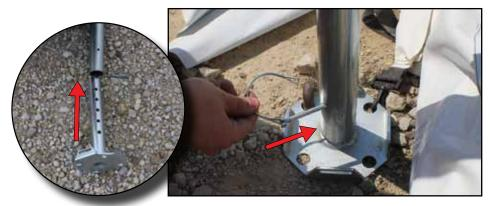
9. Lift one side of the frame up and slide the legs (Green/HT2GST80) with base plates into the bottom of the two corner fittings (F01CORHT) and pin using pin & bail (HT570). Slide the pin through the hole in the corner fitting and leg hole then connect the bail end around the pin.
