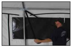
6. Remove the four middle legs with base plates and place off to the side.
