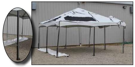
14. Layout the floor underneath the frame.
