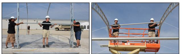
6. Assembling the wind brace supports: Wrap the tube clip (#17A) around the interior arch. The tube clip is movable to ensure the proper position. Install the wind brace support (#17) that connects the front arch to the first interior arch. The wind braces give the arch assemblies strength as a unit. Use bolt M10x30 (#30) at the end of each wind brace support to secure.
