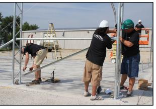
7. Install the other arch assemblies in the same manner. Overlap pinched ends of roof purlins onto same carriage bolts inside frame assembly.
