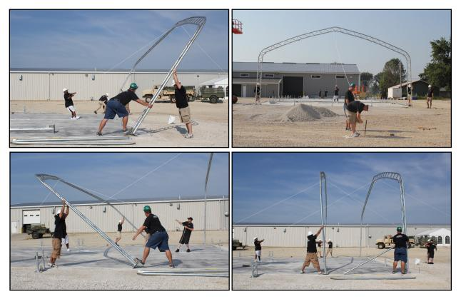
5. Assembling the roof purlins: Immediately after erecting the first arch, erect the 2nd arch in the same way. Connect the two erected arches using the roof purlin and horizontal tubes (#5). Secure the roof purlin tube into place using carriage bolts and nuts (#28A). **Note:** that the 2nd arch should be assembled with the base plate (#8A) so the wind brace support can be connected.
