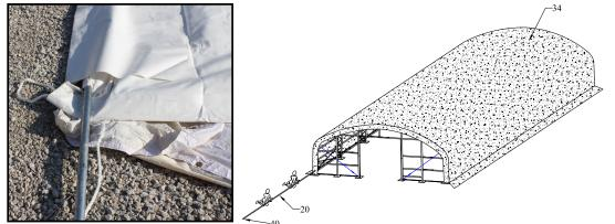
15. Make small cuts using a scissors in the roof cover pocket for the ratchet tie down strap to go through. Draw the outline of the cuts according to the position of the ratchet (#32). Cuts should be right upon the ratchets.
