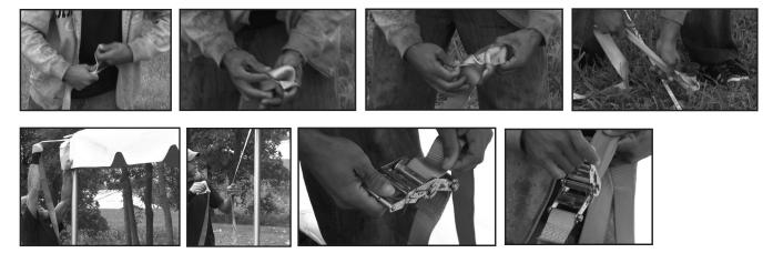
21. Make sure the legs are straight then secure the master series base plates by driving a double-headed stake through the smaller tubing on the master series base plate. Tighten all ratchet assemblies.
