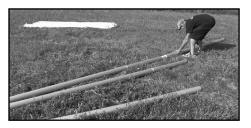
9. Insert the center pole pin through the center nipple/floor flange assembly; make sure that the pin is not caught on any part of the tent top. Lift the top using the center pole(s) and set pole at an angled position so the top is completely off the ground. Insert a tent stake into the helper hole on the center pole if available.
