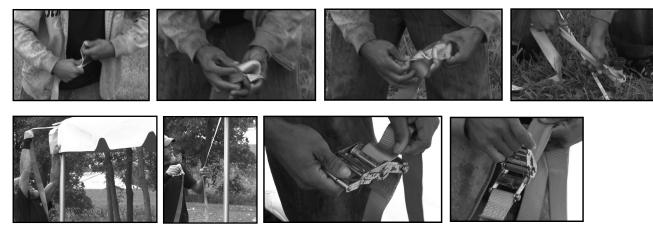
20. Make sure the legs are straight then secure the master series base plates by driving a double-headed stake through the smaller tubing on the master series base plate. Tighten all ratchet assemblies.
