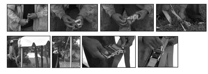
19. Make sure the legs are straight then secure the master series base plates by driving a double-headed stake through the smaller tubing on the master series base plate. Tighten all ratchet assemblies.
