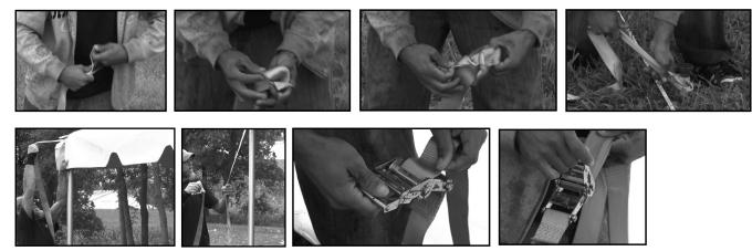
17. Make sure the legs are straight then secure the master series base plates by driving a double-headed stake through the smaller tubing on the master series base plate. Tighten all ratchet assemblies.
