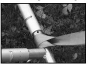
7. Roll out a drop cloth to protect the tent from dirt and abrasions next to the frame and unroll the tent top. The tent needs to be laid out in the sequence of: 20'x10' grommet end, 20'x20' midsection (x3), and 20'x10' lace end. (The midsection has a lace and grommet side; each seam requires one lace line and one grommet line for fastening.)
