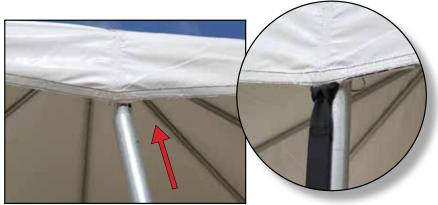
13. Locate the remaining tent top straps, 120" (300 cm) in length, and attach. Attach the loop end through the 11/2" (3.81 cm) welded D ring, run the rest of the strap through the loop and outside slot of the base plate, and pull tight.
