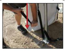
19. Locate the fourteen X-Bracing straps (HT531), 148" (370 cm) in length. On each corner and side tee fitting take the loop end through the 11/4" (3.175 cm) welded D rings on either side of the hip/rafter poles, run the rest of the strap through the loop, and pull tight.
