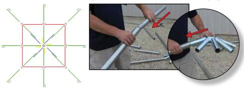
3. Take the combined hip rafter poles (Green/HT2GST80) and slide onto the remaining post slots on the 8 way crown (F048WCHT). Lining up the holes until the push pins engage.
