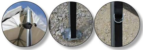
11. Lift the other side of the frame up and slide the legs with base plates into the bottom of the remaining corner fittings and pin using pin and bail.
