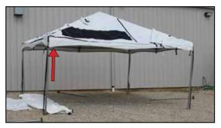
12. Put the other four legs with base plates on the bottom of all of the side tee fittings and pin with pin and bail.
