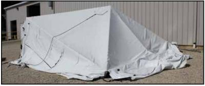
Remove the other two corner legs and base plates, place off to the side, and carefully set the frame all the way down.
