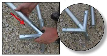
5. Locate and slide all four of the side tee fittings (F02STHT) into the hip rafter poles (Green/HT2GST80). Lining up the holes until the push pins engage.
