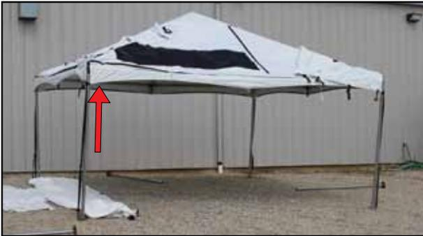
12. Put the other four legs with base plates on the bottom of all of the side tee fittings and pin with pin & bail.
