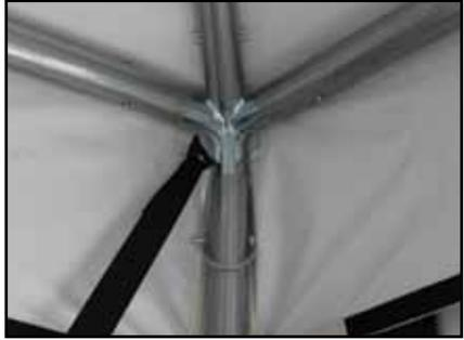
20. **NOTE:** *X-Bracing straps go on every bay except the bay with the door.* To find the door bay stand under the center of the tent facing the direction of the roof vent. The door bay is directly in front on the left.
