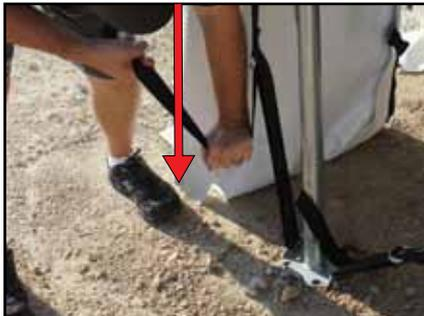
19. Locate the fourteen X-Bracing straps, 148” (370 cm) in length. On each corner and side tee fitting take the loop end through the 1¼” (3.175 cm) welded D rings on either side of the hip/rafter poles, run the rest of the strap through the loop, and pull tight.
