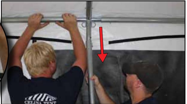
7. On one side remove both legs with base plates from the corners, place off to the side, and carefully set the frame down. **NOTE: Do not set frame on sidewalls.**
