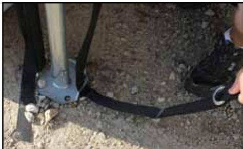
22. Tighten each strap by running the tail end of the strap through both D rings and then back through the lower D ring. Pull the tail end downward to tighten. Use a foot if necessary to tighten the straps.
