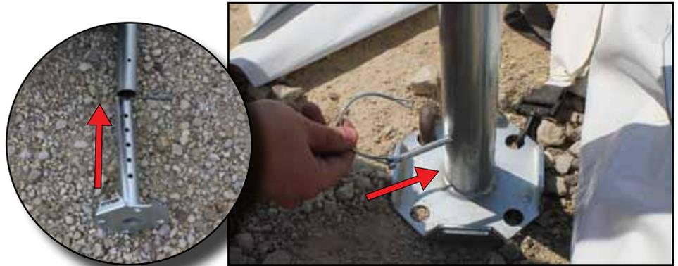
9. Lift one side of the frame up and slide the legs (Green/ HT2GST80) with base plates into the bottom of the two corner fittings (F01CORHT) and pin using pin & bail (HT570). Slide the pin through the hole in the corner fitting and leg hole then connect the bail end around the pin.
