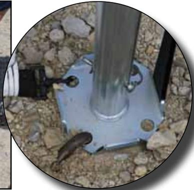
17. Take the ends of the straps down through the outside slot on each base plate.
