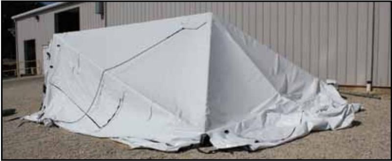
8. Remove the other two corner legs and base plates, place off to the side, and carefully set the frame all the way down. **NOTE: Do not set frame on sidewalls.**
