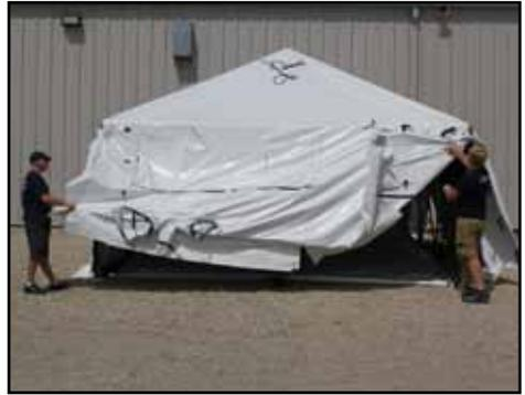
24. Close all corners by connecting all of the side release buckles and tightening. ***NOTE: Door must be closed prior to tightening side release buckles.***
