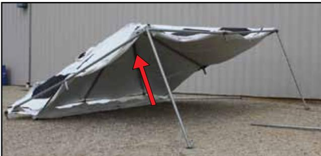
10. Locate the corner tent top straps, 120" (300 cm) in length (HT531). To attach the tent top strap on a corner take the loop end through both 1½" (3.81 cm) welded D rings on each side, run the rest of the strap through the loop, and pull tight. To reattach a removed tent top strap on a side take the loop end through the 1½" (3.81 cm) welded D ring, run the rest of the strap through the loop and outside slot of the base plate, and pull tight.
