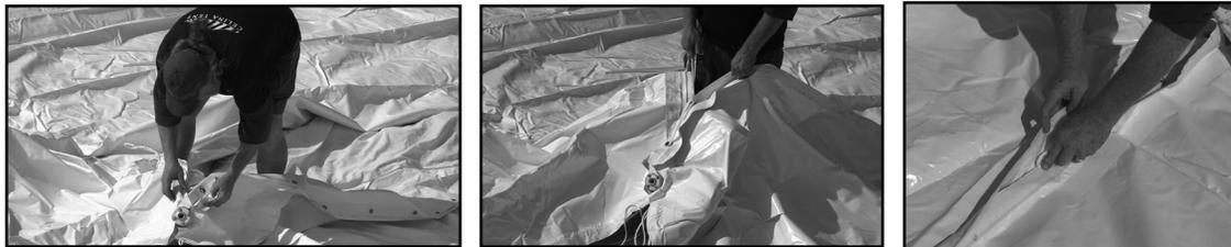
3. Attach the tie back straps to the plates on the tent top. Make sure the two center holes in the plates are aligned for the side poles, while hooking the tie back straps to the larger holes towards the edge of the plates.
