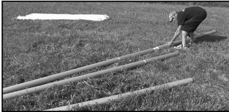
9. Insert the center pole pin through the center nipple/floor flange assembly; make sure that the pin is not caught on any part of the tent top. Lift the top using the center poles and set pole at an angled position so the top is completely off the ground. Insert a tent stake into the helper hole on the center pole if available.
