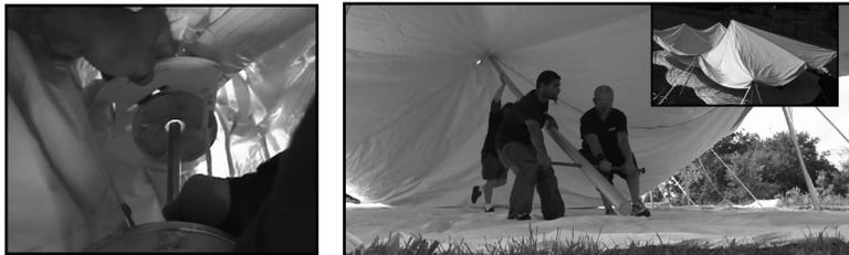
10. Tie off the jump rope attached to the center pole locations (eye level: 5-6 feet).
