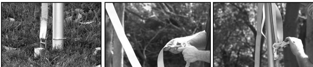
16. Repeat with the other side of the tent. When finished with the corner legs, install all other legs at side tee fitting locations. Pull the anchoring devices (ratchet buckle strap) through the tops of the hook and loop extensions on the tent top to provide access to the stakes.
