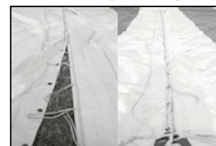
9. Pull the tent top over the frame, lifting up on the fabric or "flapping" it to create a cushion of air. Make sure the tent top is centered from all sides.
