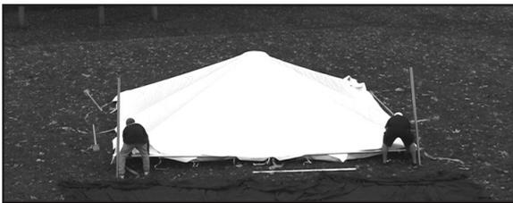
11. Connect the O-ring of the master series ratchet buckle (C) to the base plate hook mounted on the small tubing of the base plate. Feed the master series loop strap (D) attached to the tent top through the reel bars slot of the ratchet (ratchet buckle needs to have handle facing upward at all times) and pull the strap back towards the tent approximately 1 ½ feet. Hold the strap at this point with one hand and begin to crank the ratchet handle back and forth.
