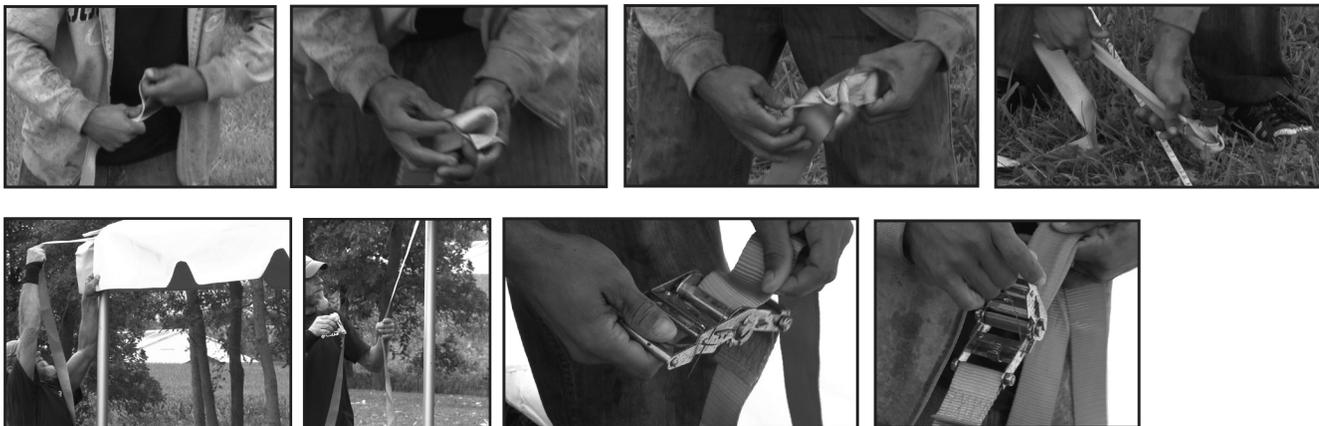
15. Make sure the legs are straight then secure the master series base plates by driving a double-headed stake through the smaller tubing on the master series base plate. Tighten all ratchet assemblies.
