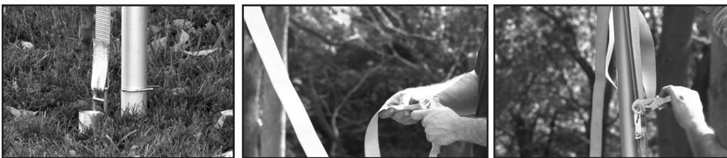
12. Repeat with the other side of the tent. When finished with the corner legs, install all other legs at side tee fitting locations. Pull the anchoring devices (ratchet buckle strap) through the tops of the hook and loop extensions on the tent top to provide access to the stakes.
