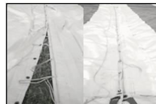
8. Pull the tent top over the frame, lifting up on the fabric or “flapping” it to create a cushion of air.
