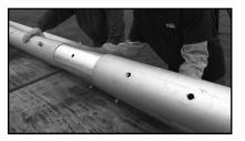
9. Insert the center pole pin through the center nipple/floor flange assembly; make sure that the pin is not caught on any part of the tent top. Lift the top using the center pole(s) and set pole at an angled position so the top is completely off the ground. Insert a tent stake into the helper hole on the center pole if available.
