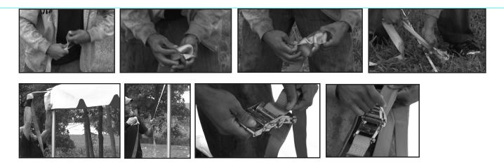
18. Make sure the legs are straight then secure the master series base plates by driving a double-headed stake through the smaller tubing on the master series base plate. Tighten all ratchet assemblies.
