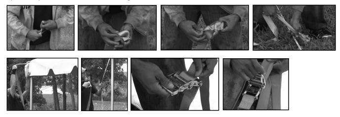
16. Make sure the legs are straight then secure the master series base plates by driving a double-headed stake through the smaller tubing on the master series base plate. Tighten all ratchet assemblies.
