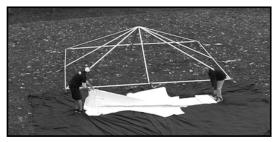
6. The tent needs to be laid out in the sequence of: 15'x7.5' grommet end and 15'x7.5' lace end.
